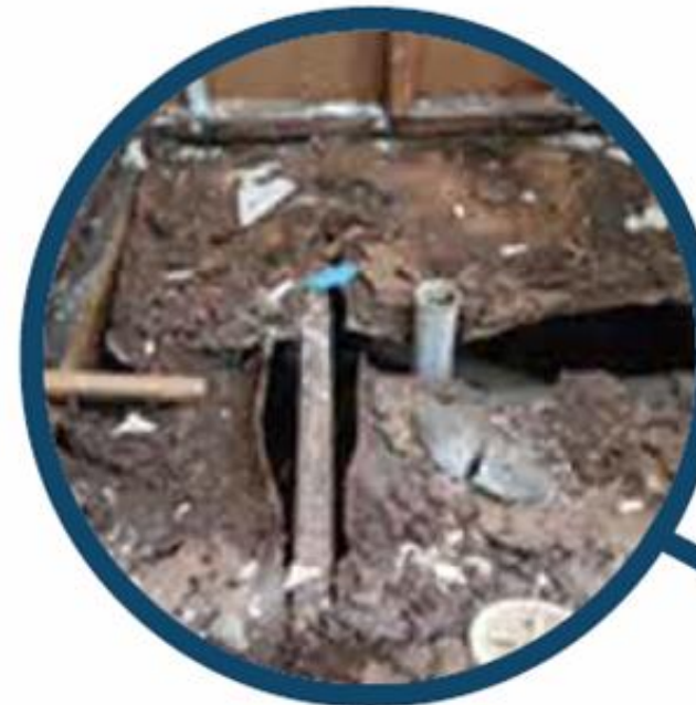
FAILED WATERPROOFING MEMBRANES IN SHOWER RECESSES
