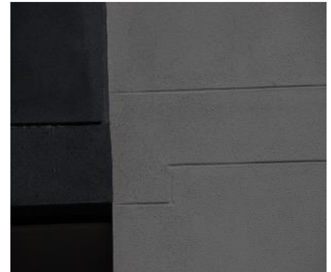
FIGURE 4.2 SLIP JOINT
