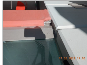
Photograph 5 - Building 1, Unit 306, Balcony Overflow External Close-up
