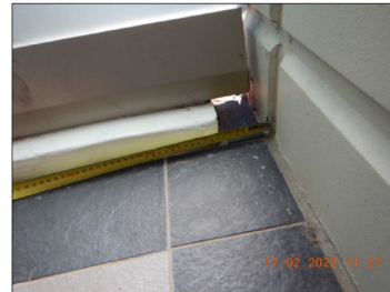
Photograph 4 - Building 1, Unit 306, Balcony Overflow Width (approx. 70mm x 45mm)
