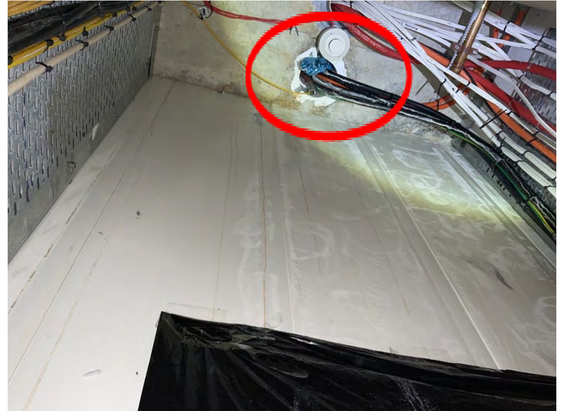
Unprotected fire penetration or opening
