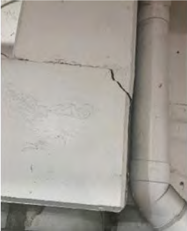
Cracking in concrete
