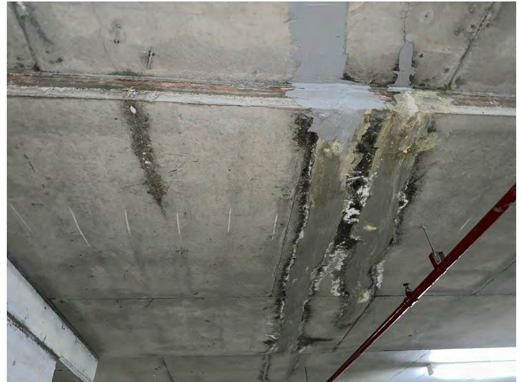
Cracking in concrete
