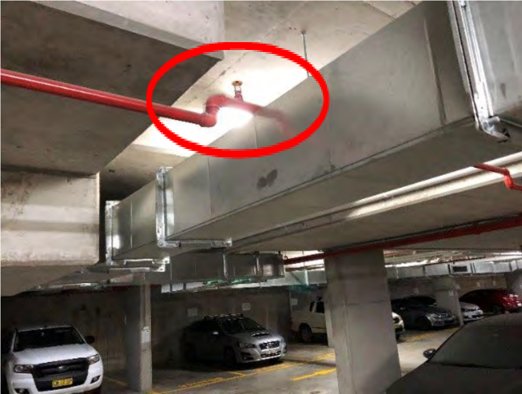
Fire sprinkler obstruction
